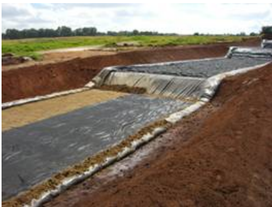
Figure 1: Construction of cascade system
