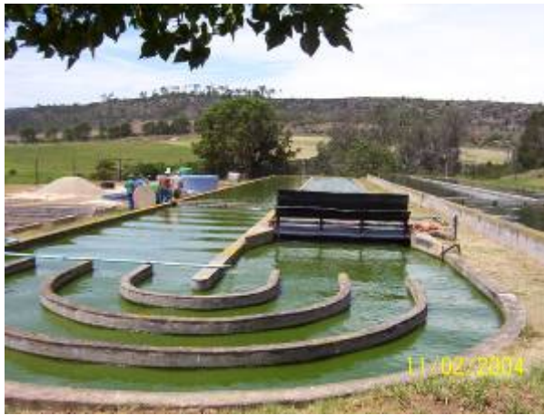
Figure 2 One of the High Rate Algal Ponds at the EBRU field station, in which algae grows, taking in nutrients and raising the pH
