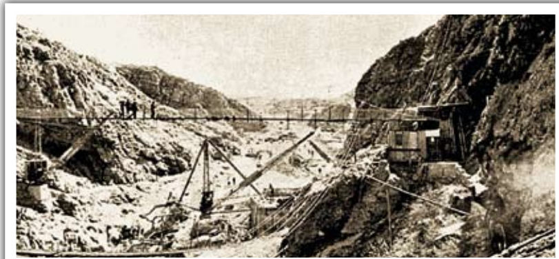
Cable way at Hartbeespoort Dam during the construction of the foundations, 1922.
