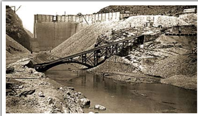
Hartbeespoort Dam during construction of the wall.
