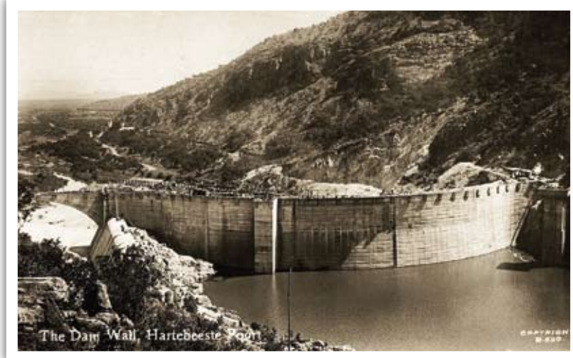
Completed Hartbeespoort Dam.
